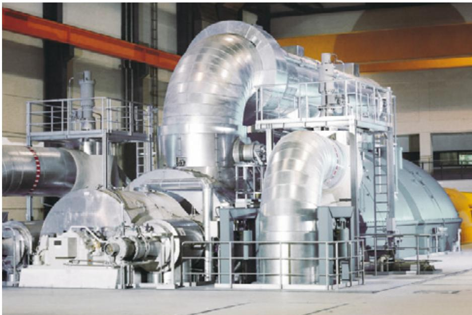
874 MW steam turbine at Schwarze Pumpe lignite-fired power plant
